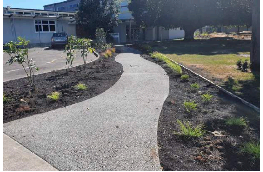
Our newly completed path to the hall.
